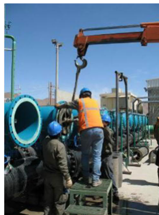
Figure 18: Supporting the internal assembly
