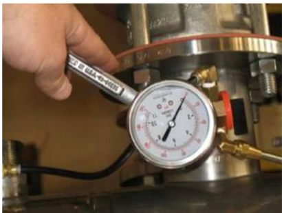
Figure 31: Removal of pressure gauge
