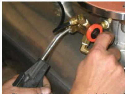
Figure 32: Blowing out air lines
