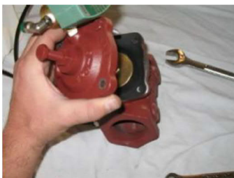
Figure 41: Removal of diaphragm cover plate
