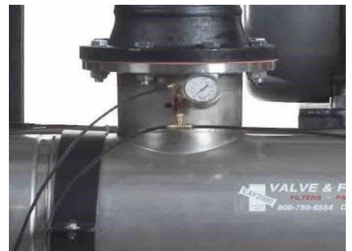
Figure 6: 3-Position manual valve and pressure gauge
