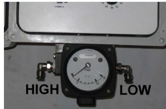
Figure 7: High- & low-pressure ports on the DP switch/gauge
