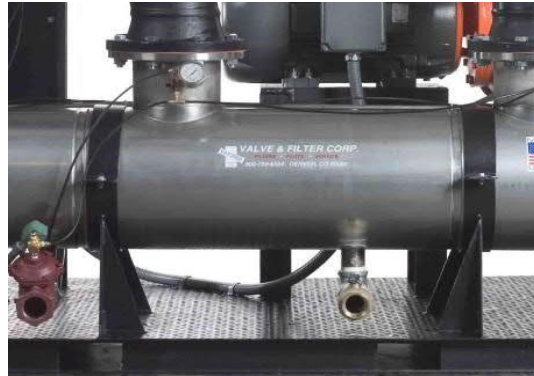
Figure 2: Saddle type filter support
