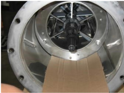
Figure 14: Covering the inlet line
