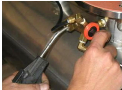
Figure 32: Blowing out air lines
