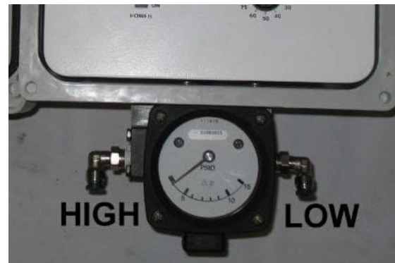
Figure 7: High- & low-pressure ports on the DP switch/gauge
