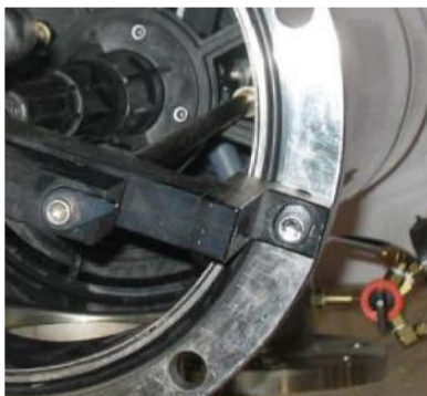
Figure 17: Puller shown bolted to the lid flange
