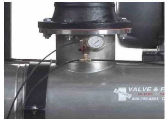
Figure 6: 3-Position manual valve and pressure gauge
