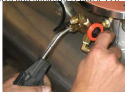
Figure 40: Blowing out air lines
