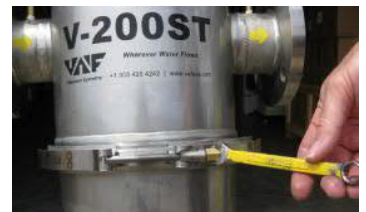
Figure 6: Unbolt clamp
