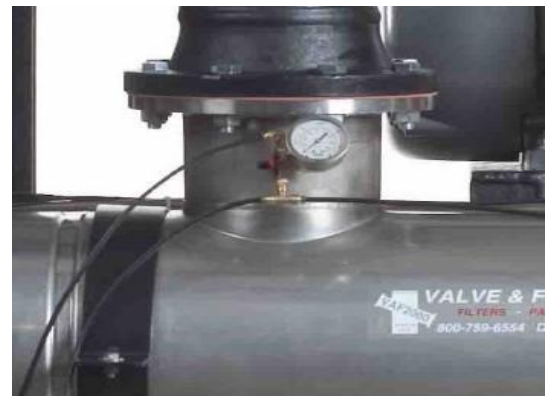
Figure 6: 3-Position manual valve and pressure gauge
