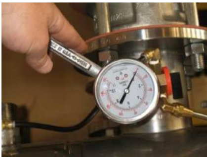
Figure 31: Removal of pressure gauge
