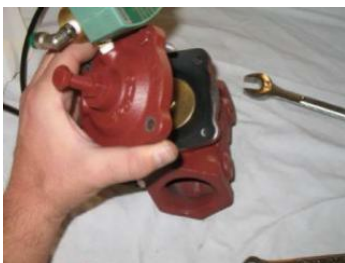
Figure 41: Removal of diaphragm cover plate
