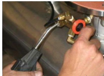
Figure 32: Blowing out air lines
