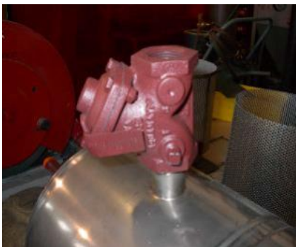
Figure 33: Flush valve
